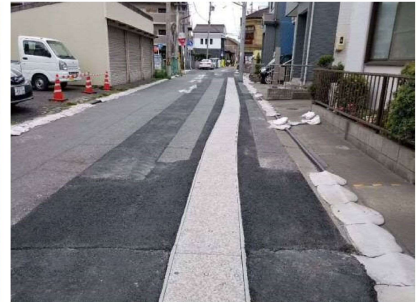
据付完了 (As 舗装) (曲線部施工状況)
