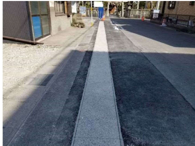
復旧完了 (As 舗装)
