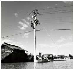
Restored distribution line after Typhoon Isewan (1959)
