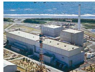
Hamaoka Nuclear Power Station Unit 1 (1976)
