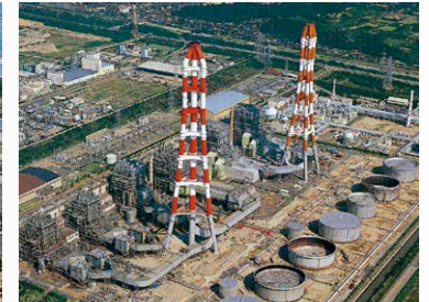
Chita Thermal Power Station Units 5 and 6 (1978)
