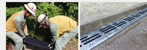
Installing covers for gutters
