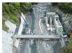
Abekawa Hydro Power Plant (Embankment construction status)
