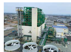
Yonago Biomass Power Plant (Operation commenced in April 2022)
