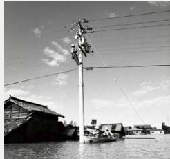
Restored distribution line after Typhoon Isewan (1959)
