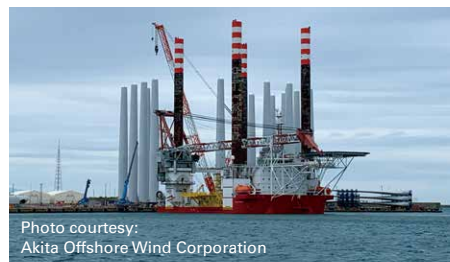
Preparing for windmill installation (Akita Port)
