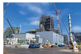
Kamisu Biomass Power Plant (Construction work status)
