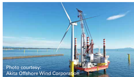
A windmill installation by self elevating platform (Noshiro Port)
