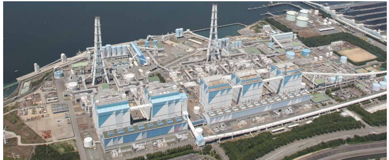
Hekinan Thermal Power Station undertaking a demonstration project for ammonia co-firing
