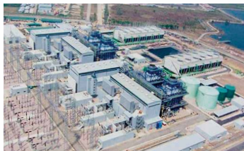
Ratchaburi gas thermal IPP (independent power producer) project in Thailand (2008)
