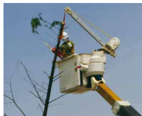
Tree-felling training assuming damage to power distribution equipment caused by fallen trees.
