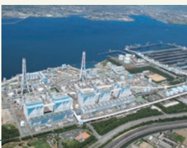
Hekinan Thermal Power Station (1991)
