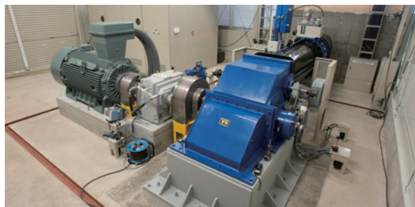
Akigami Hydroelectric Power Station (power generator) Power generation scale: 290 kW small-scale hydropower station that uses maintenance flow*
