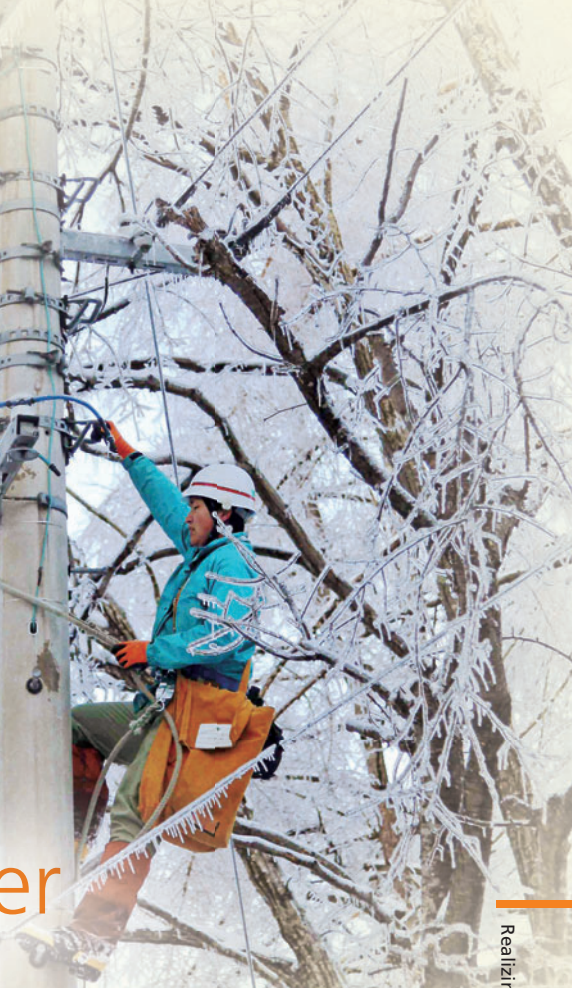
Restoration work during a snowstorm
