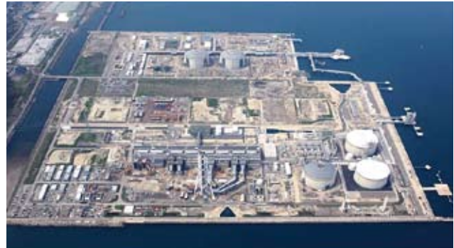
Joetsu Thermal Power Station: Unit No. 1-1 started operation in July 2012
