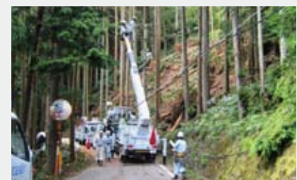
Restoration work underway by Toenec's employees
