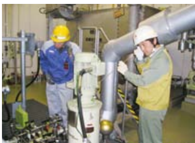
Inspection at Insulation Oil Recycling Center
