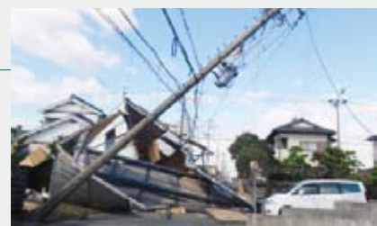
Damage caused by Typhoon #15
