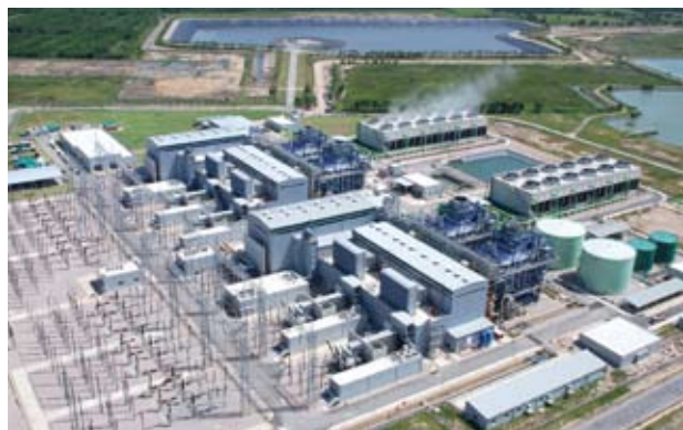
In Thailand, we invest in gas thermal power generation and provide technical support for power station operation and maintenance (Thailand Ratchaburi Gas Thermal Power Generation Project).
