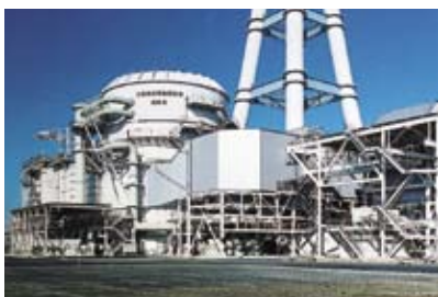
Fuel-gas desulfurization facility at Hekinan Thermal Power Station
