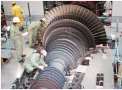
An inspection at the Shin-Nagoya Thermal Power Station
