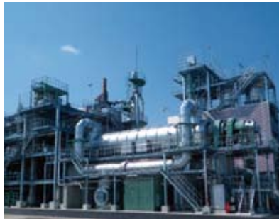
Sewage-sludge-to-fuel conversion facility in the Kinuura East Purification Center
