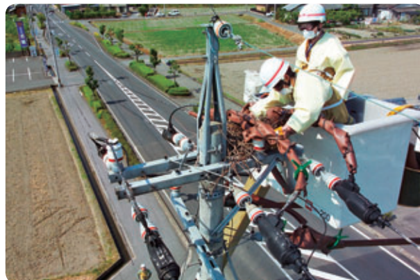
Crow's nest removal work
