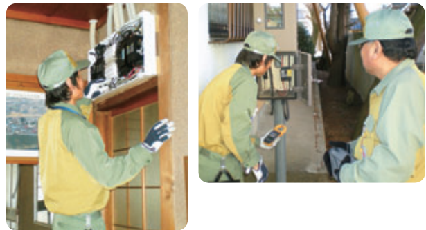
Checking wiring at cultural properties like Yakushiji Temple and Kawano Sainyubo in collaboration with the Kakamigahara City fire department and city government (Kakamigahara Customer Service Office, Gifu Regional Office)
