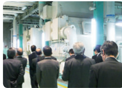
Observing the Centrair Japan International Airport Energy Center
