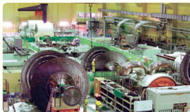
Unit No. 5 low-pressure turbine being replaced
