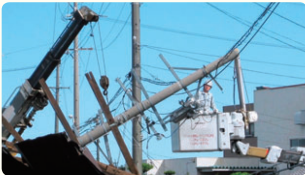
Recovery work performed by TOENEC employee (Tsu City, Mie Prefecture)
