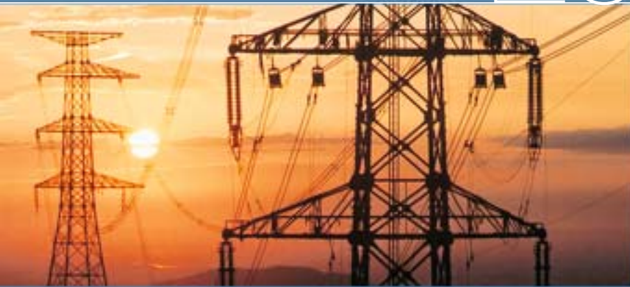
The 275-kV Kota Shin-Mikawa Line under construction (operation started May 2006)
