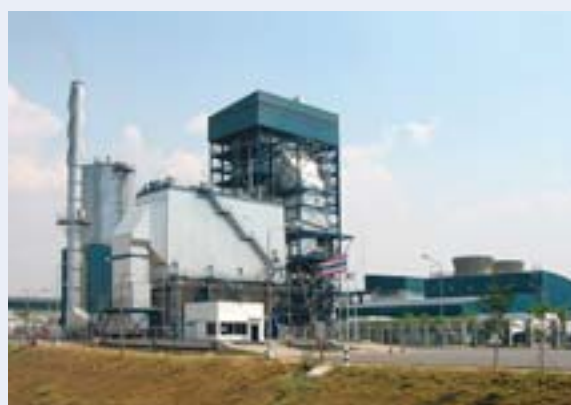
A rice-chaff-fueled power generation facility in Thailand
