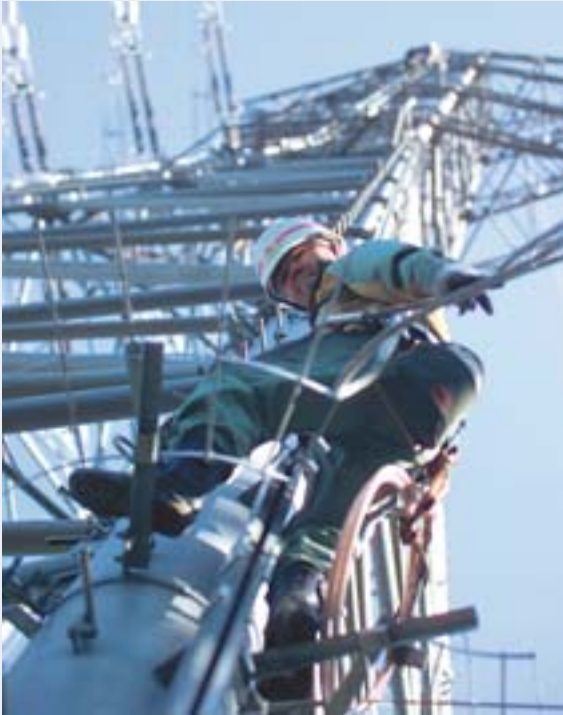
Quality inspection of the transmission tower
