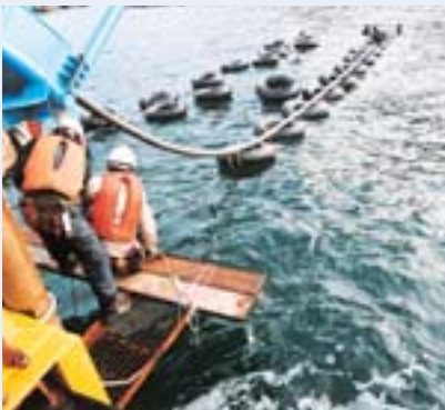
Laying an 8-km undersea cable to Kamijima Island (Toba city, Mie Prefecture) in order to switch power supply from remote-island generator to power grid. The island began drawing power from the power grid in June 2005.
