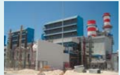
Part of the Qatari power-generation facilities went online in May 2006
