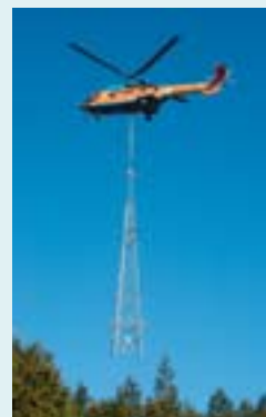
Tower carried to level ground by a helicopter
