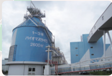
Woody Biomass Fuel Mixed Combustion Facility (Hekinan Thermal Power Station)
