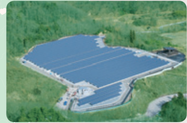
Mega Solar Iida
