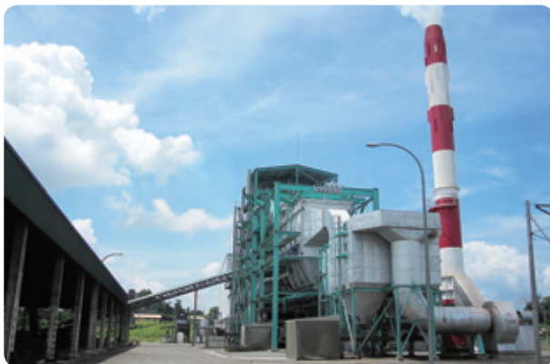
Oil palm empty fruit bunch power generation project in Malaysia
